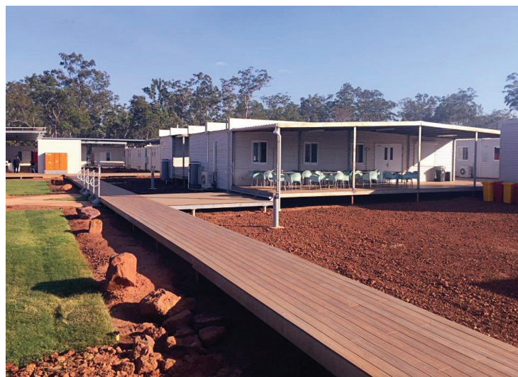
Accommodation and recreation room
